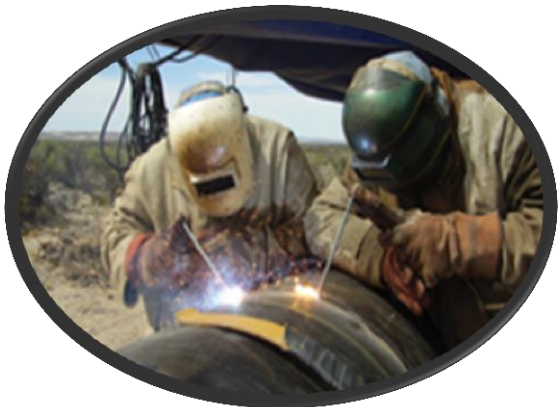
FORMATION OF WELDERS WITH SMAW PROCESS
