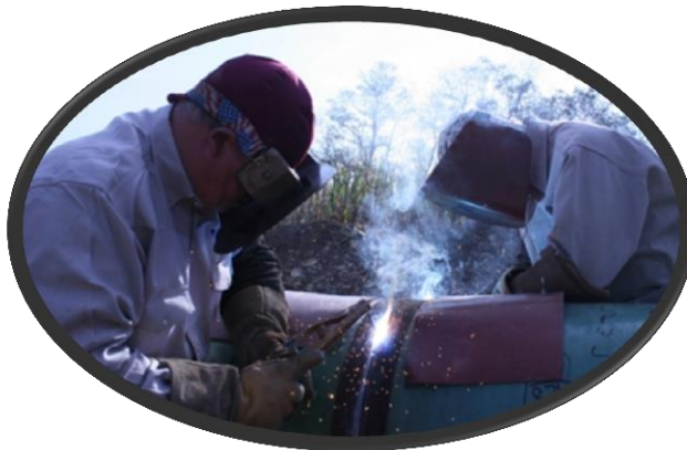
PIPELINE WELDING WITH SMAW PROCESS
